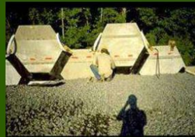
Filter Fabric Placed Over Openings Between Hexagonal Panels
