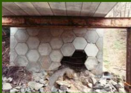
Abutment Failure (Blow-Out) Due to Built-Up Hydrostatic Pressure
