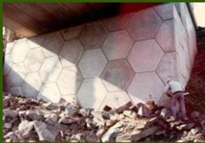
Filter Fabric Placed Over Openings Between Hexagonal Panels
