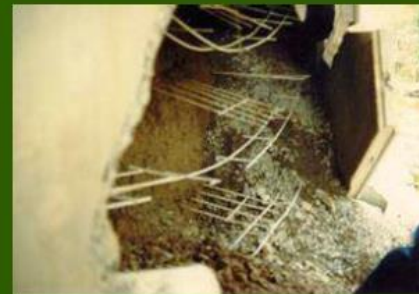
Abutment Failure (Blow-Out) Due to Built-Up Hydrostatic Pressure
