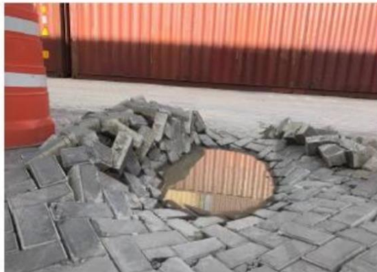
Picture 1 General shear strength failure type observed in segment 1.1.
