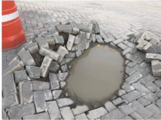
Picture 1 General shear strength failure type observed in segment 1.1.
